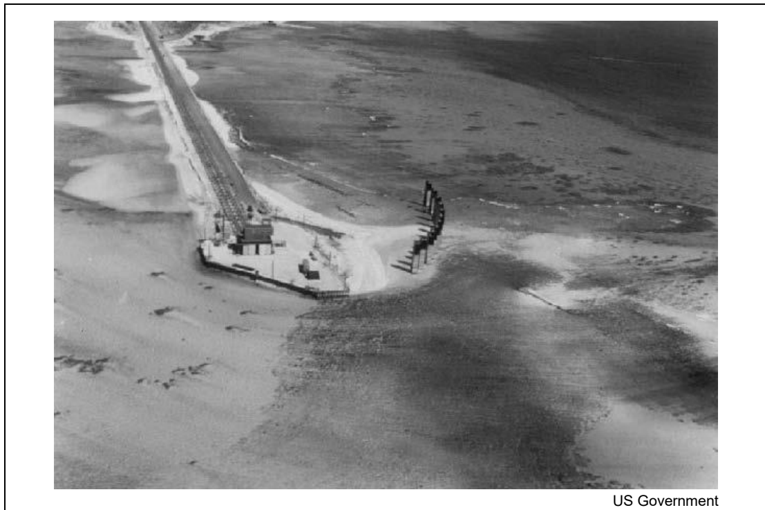
Figure 1-12. BRAVO shot site showing the causeway with vacuum line-of-sight pipes connected to the shot cab
