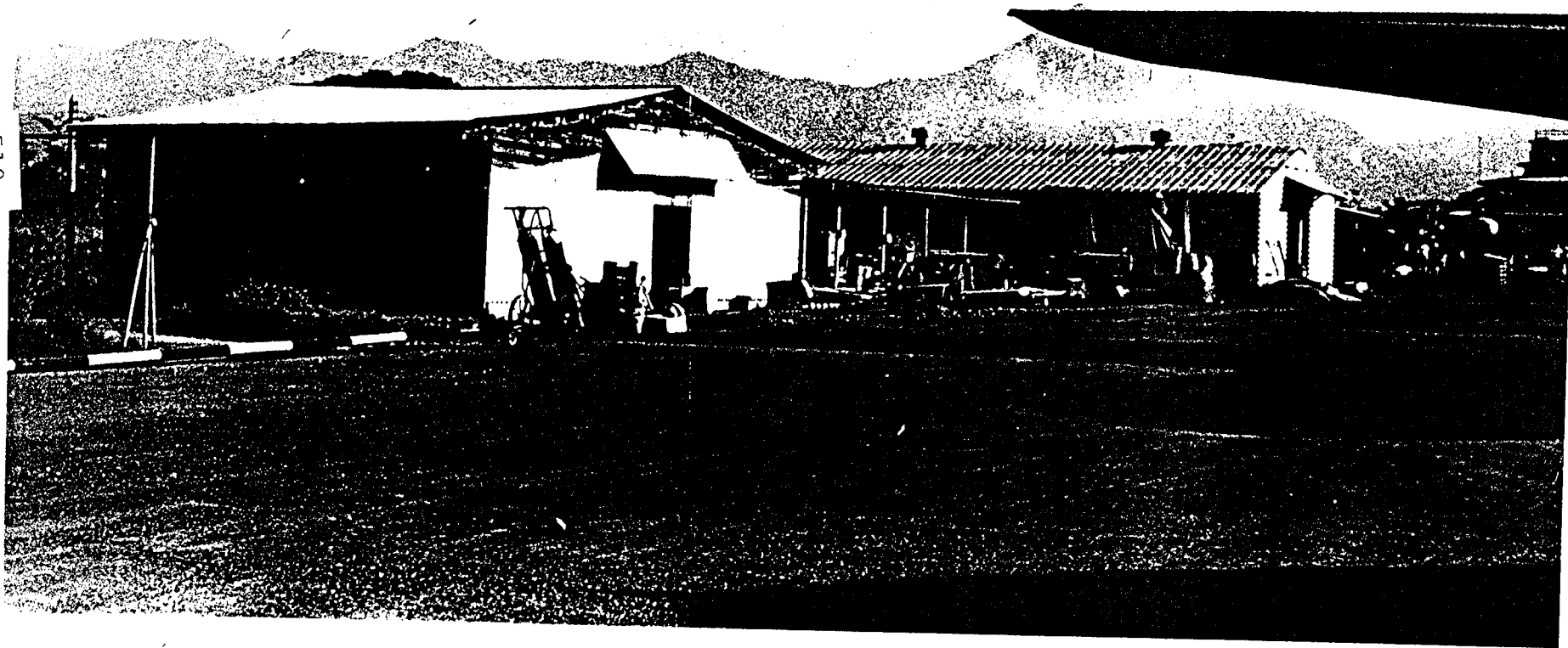
FIGURE 4 RETALHULEU SERVICE AND MAINTENANCE AREA
