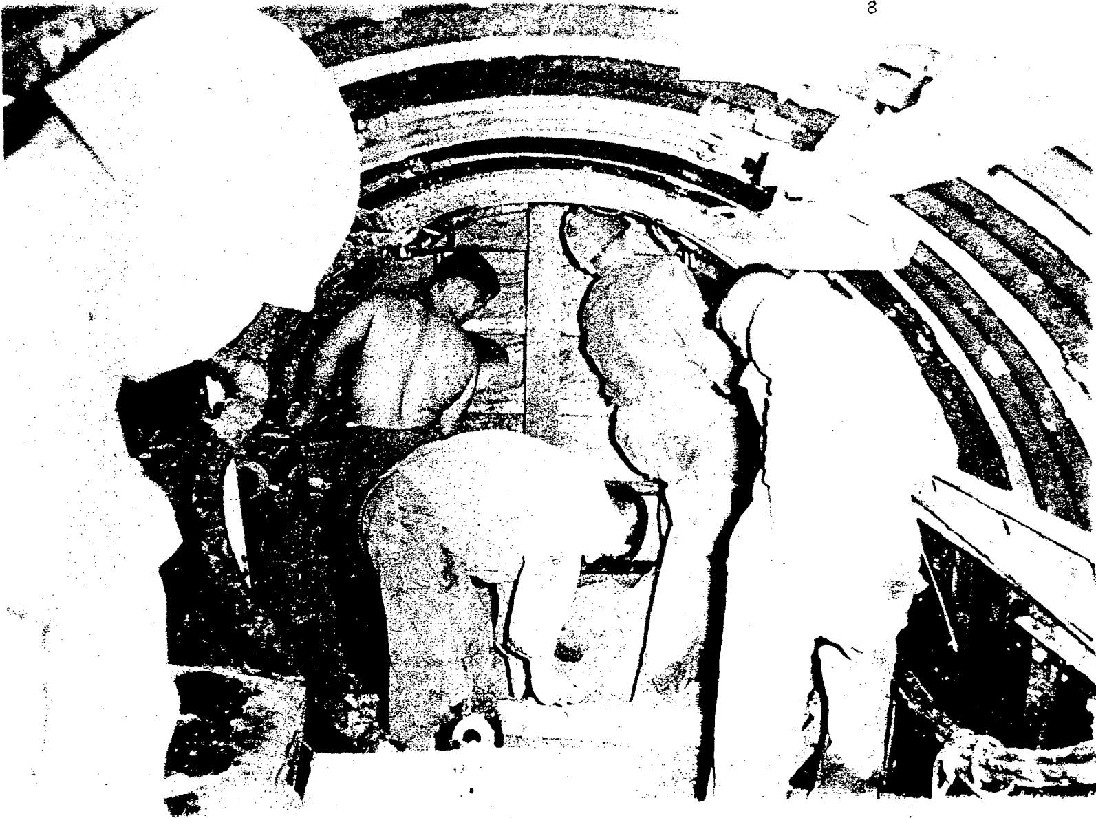
Figure 8 - Excavating Using the Blinds
