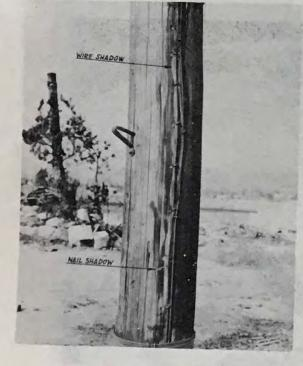
Figure 7 "SHADOWING" EFFECT OF WIRE ON TELEPHONE POLE (Note sharp line of shielding by nail near bottom.)
