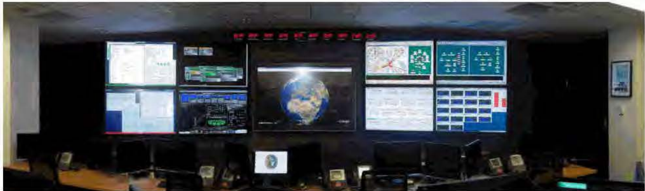
Figure 1-14. JBC-P Network Operations Center
